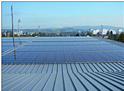
204.4 kWp Bossard Arena Zug
