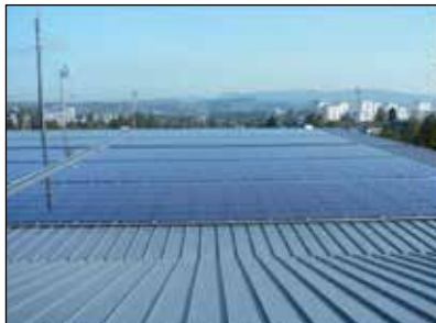
204.4 kWp Bossard Arena Zug
