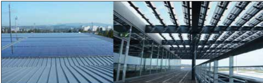
204.4 kWp Bossard Arena Zug
